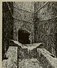
At the top of the Grand Gallery lies a huge stone step, 6 feet wide, 3 feet high, which blocks the Ascending Passage and forms a platform 8 feet deep, now badly chipped and worn.
