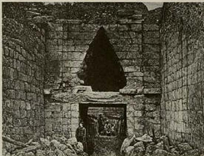
The so-called Treasury of Atreus at Mycenae built into a mound with corbeled roofing similar to the Maes-Howe mound.
