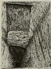
The granite plug in the ceiling, halfway down the descending passage, was of very hard quartz, mica and feldspar, which blunted the Arabs' chisels.
