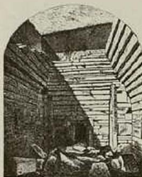
The main chamber in Maes-Howe, showing corbelled monoliths which could be closed at the top by a single movable slab. The jointing in this prehistoric masterpiece rivals that of the Great Pyramid.
