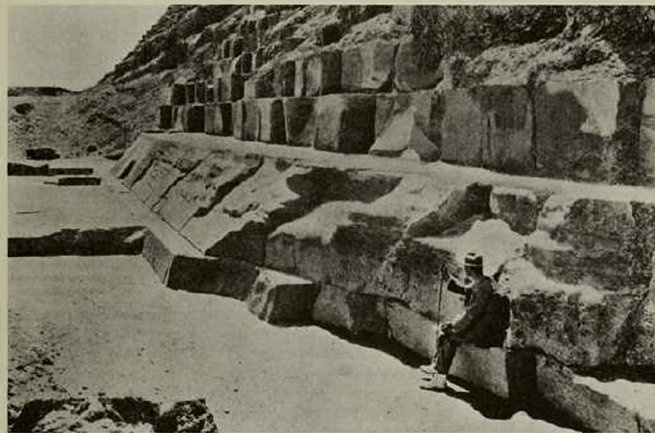
The casing stones of the Great Pyramid (looking east), showing the platform on which they rest, the pavement in front, and the leveled natural rock.
