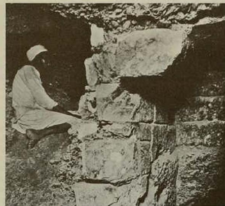
Grotto showing walls of the well shaft built out of masonry from the level of the Grotto to the first course of masonry of the Pyramid.
