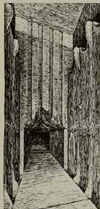
Beyond the Great Step there stretches another low, level passage 41 inches (or 2 cubits) square. A third of the way along this passage, it rises and widens into a sort of antechamber, the south, east and west walls of which are no longer of polished limestone but of polished red granite.
