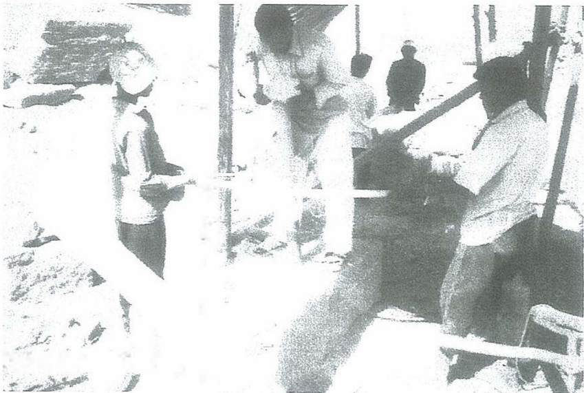
FIGURE 2. Egyptian workers drilling rose granite, with a flat-ended copper tube and dry sand abrasive. Two workers are using the stone-weighted saw in the background.
