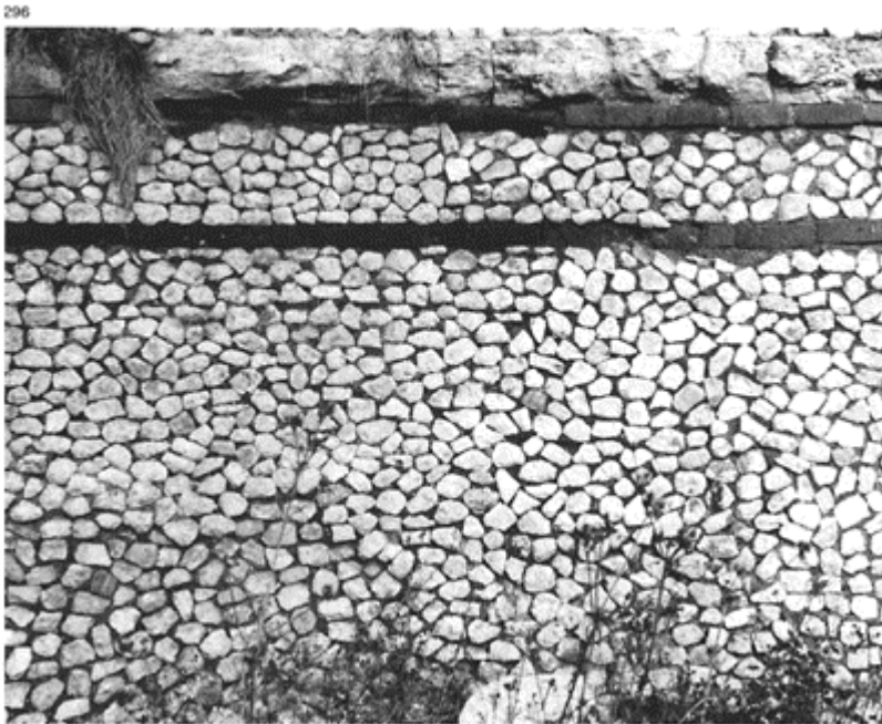
296 Temple of Fortuna at Palestrina (end of the second century BC). A facing of opus incertum with horizontal courses made of tufa rubble.
