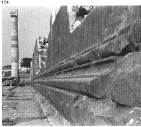
174 The Temple of Apollo at Didyma, near Miletus, despite its considerable size (118×60m), has an optical correction curve. This perfectionism led to its remaining unfinished after more than four and a half centuries of frequently interrupted construction work (from 332BC to AD 130).
