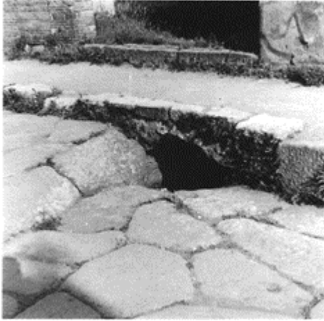
612 The mouth of a drain in the underground network at Pompeii.
