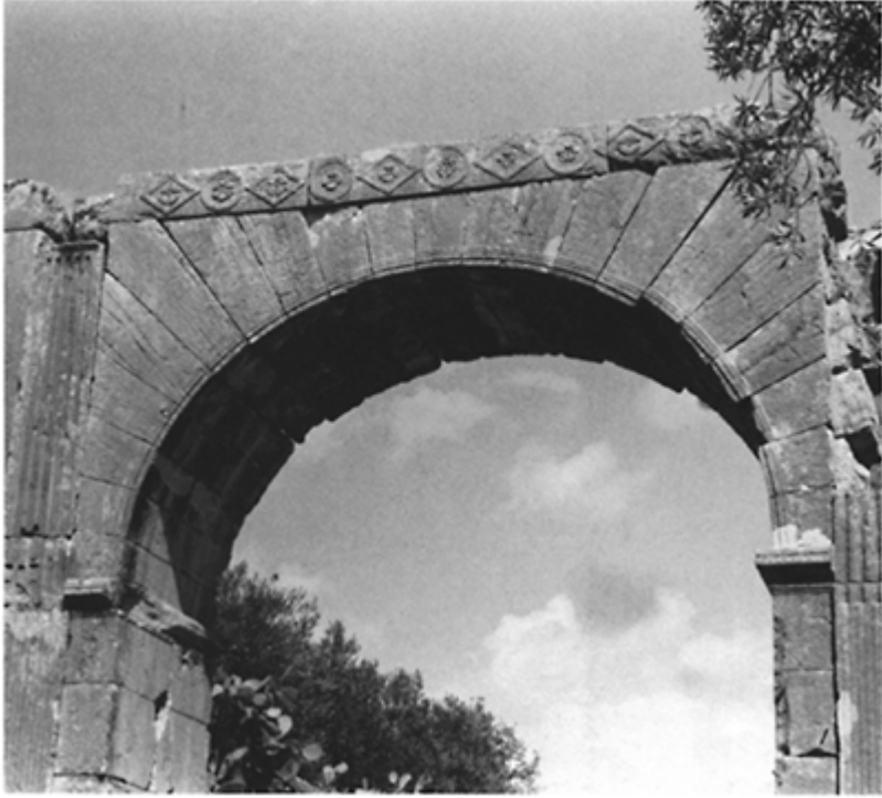
407 The Arch of Alexander Severus at Thugga (Dougga), c. 230. The extrados lines of the archstones form right angles aligned on the pilasters of the framework and a crowning band.
