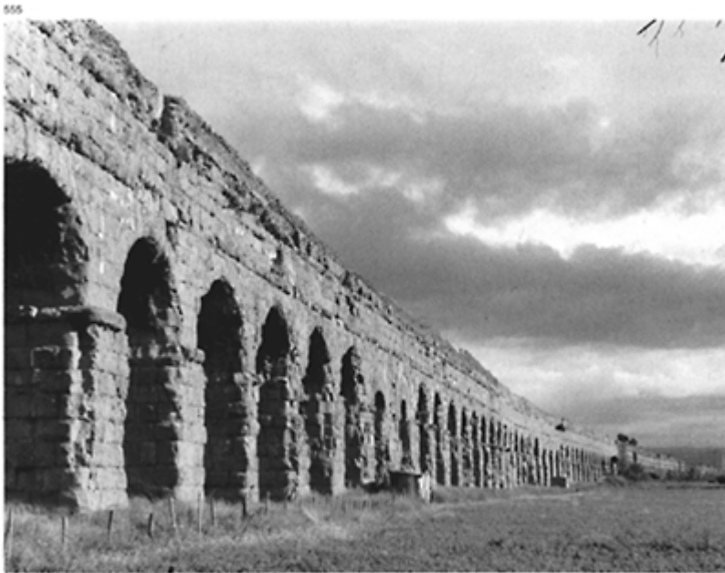
555 The impressive arcaded section of the raised stretch of the Aqua Claudia in the Roman campagna. Built from 38 to 52, this aqueduct runs for 68km, 15 of them raised. Its daily capacity was 184, 280m 3 . Later the Anio Novus was
