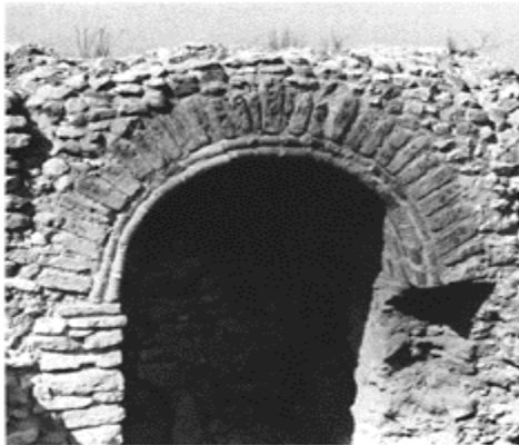
423 An arch on permanent coffering made up of a double row of ceramic cylinders. Baths at Sbeitla (Sufetula).
