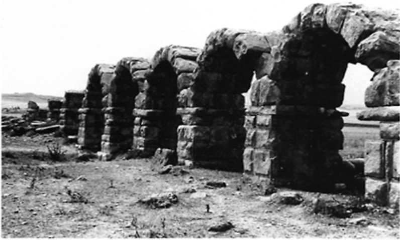
562 The massive arcaded section made of rusticated stone blocks of the aqueduct of Mactaris (Maktar) in Tunisia. Here a projecting cornice was used to support the centring.
