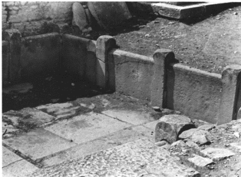
601 A public fountain at Thugga. The enormous basin is edged with slabs fitted into grooved pillars; the joints were then filled in with mortar, here partially preserved.
