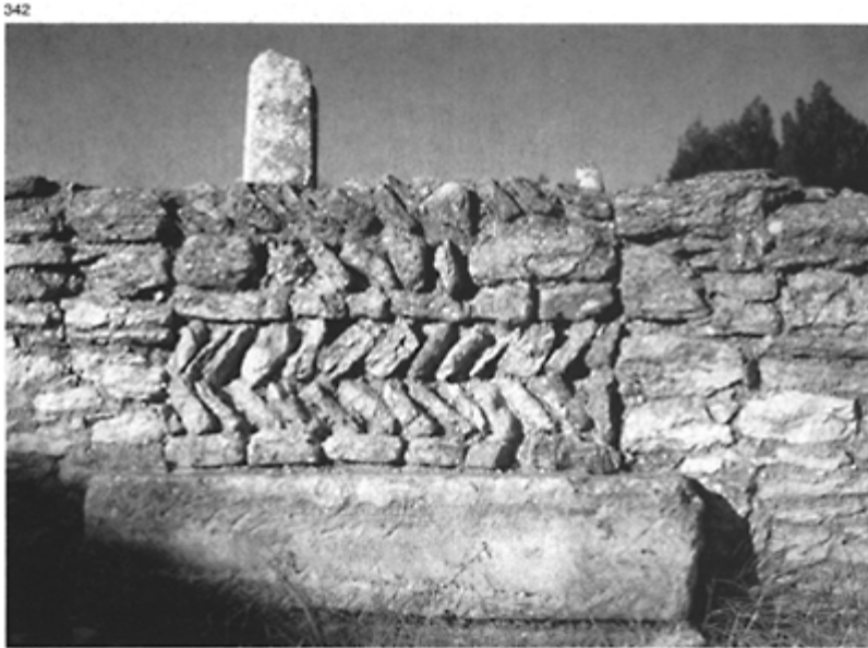
342 Walled up doorway with rough masonry of opus spicatum , at the House of the Antes at Glanum.
