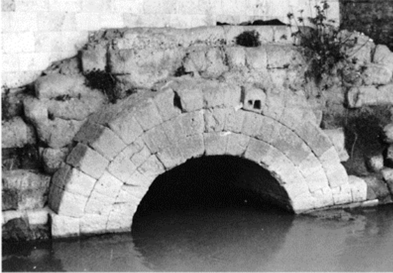
377 The outflow of the Cloaca Maxima into the Tiber, at the level of the Forum Boarium . The crown of the arch is made up of three rows of short voussoirs. The date of its construction is estimated to be the beginning of the first century BC.
