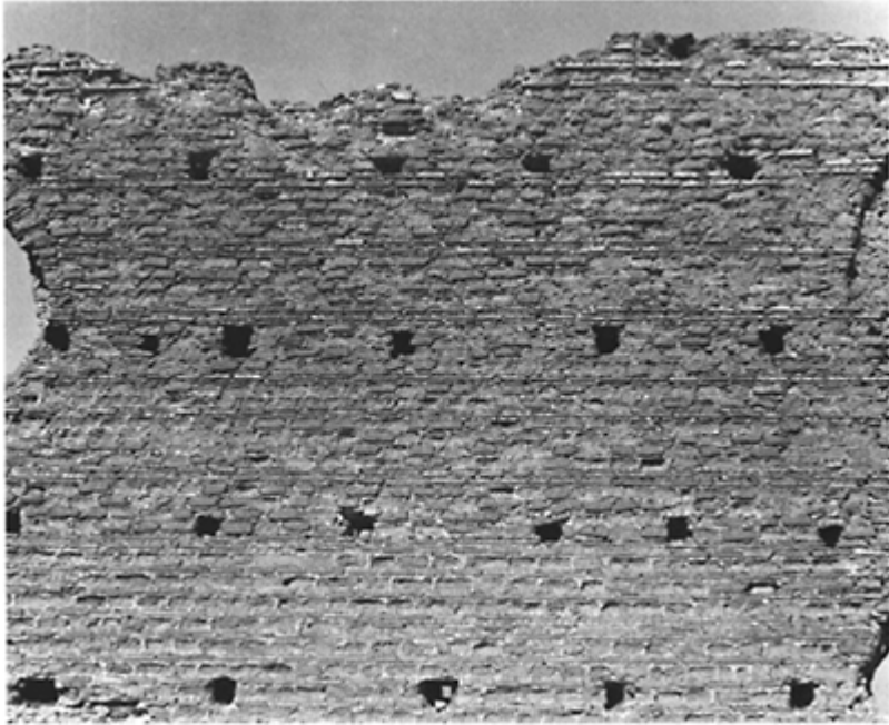
184 Transverse putlog holes in the aqueduct of the ville dei Sette Bassi ( via Latina ; c. 140)
