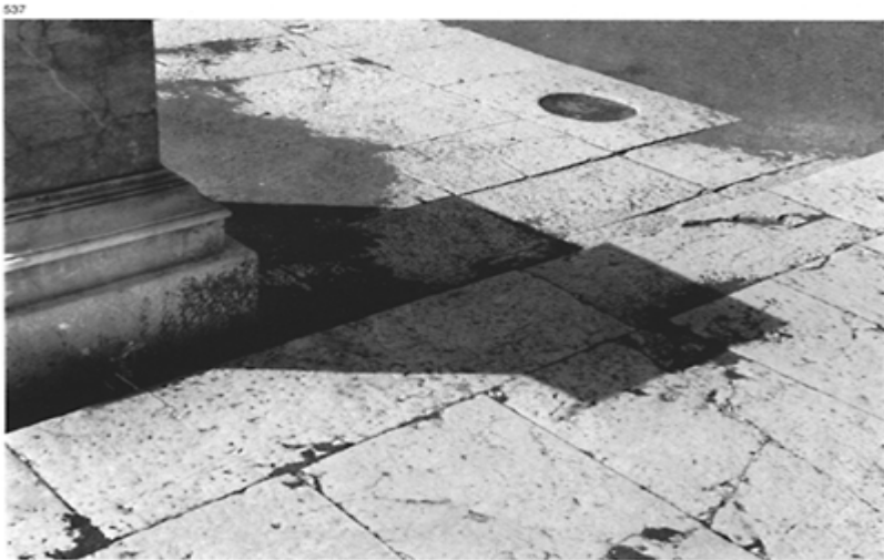
537 Thin limestone tiles in a regular rectangular pattern in an area reserved for pedestrians: the forum at Pompeii.
