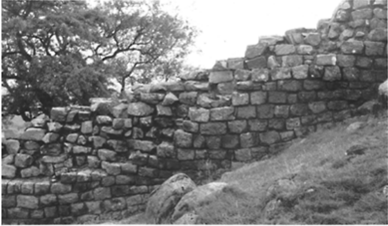
328 Section of Hadrian's Wall on a steep slope where the facing blocks are arranged in horizontal courses (c. 128).
