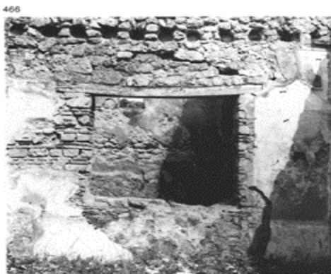
466 Housings for joists used in their natural circular shape and enclosed in the masonry. Pompeii, IX, 6, e.
