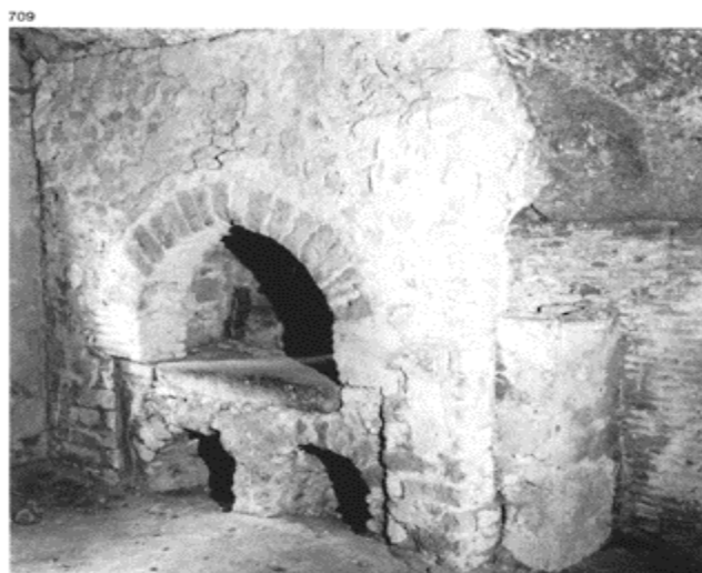
709 A kitchen installed in the basement at the House of the Centenary (IX, 8, 6); the bread oven also provided heating for the caldarium .
