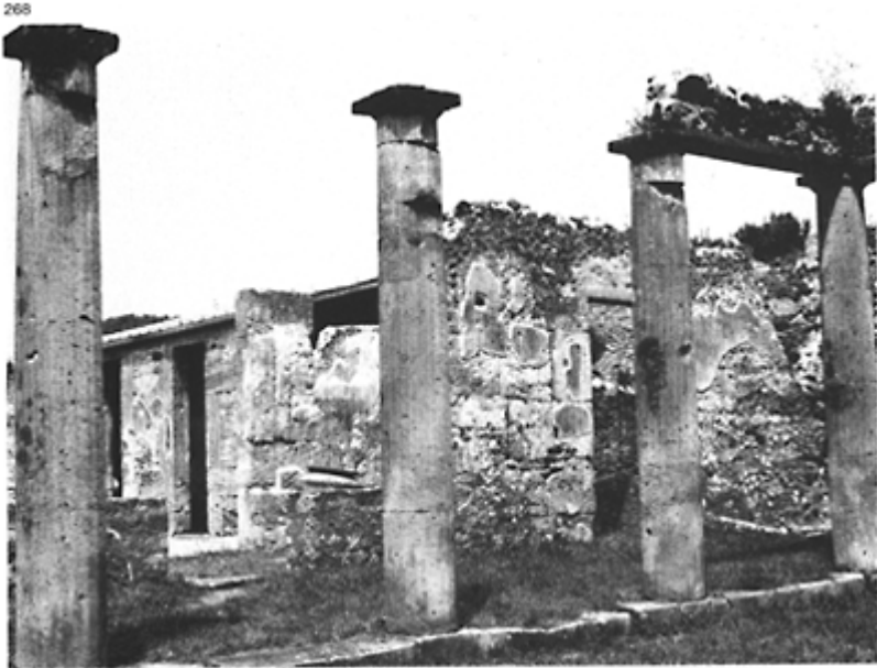
268 Peristyle colonnade of volcanic tufa; Doric order without a base, Pompeii, House of Obelius Firmus, Samnite period.
