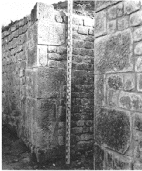
323 Amphitheatre of Senlis (first century). Facing of opus vittatum , with quoins of ashlar.
