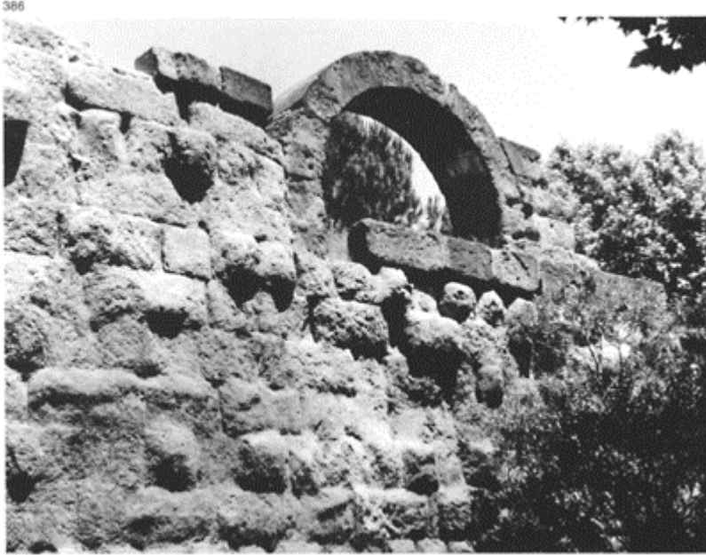
386 An opening for an artillery piece built into the Servian Wall, Rome around 90BC.
