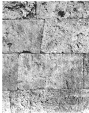
244 Walls of Pompeii. Second phase. Note the curvilinear joints from the cut of a saw.
