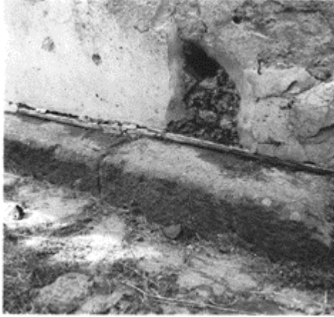
605 Lead piping from the temporary water supply network installed at Pompeii after 62. (VII, 12, 23.)
