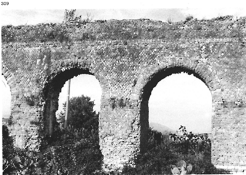
309 Aqueduct of Minturno ( Minturnae ). Masonry bonded with lime mortar with reticulate facings, the quoins and arch crowns made of small blocks. Augustan period.
