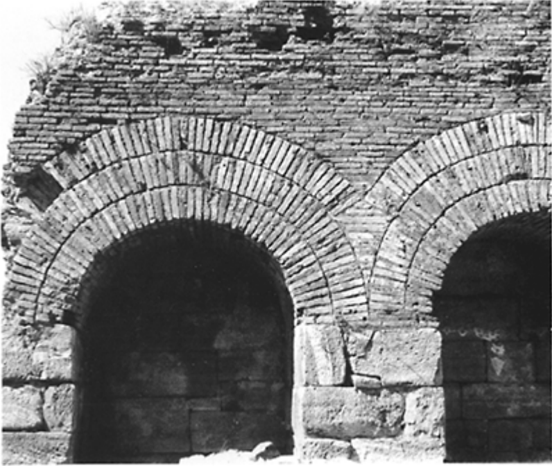
431 Niche arches at the Harbour Baths at Ephesus, made up of triple rows of bricks, built in the second century and restored under Constantine II in the fourth century.
