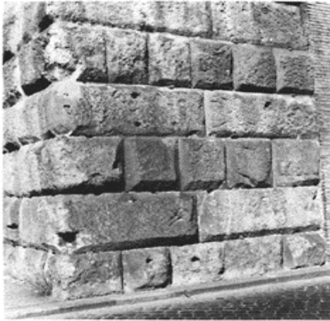
252 Regularly alternating courses of stretchers and headers on the aqua Claudia (38 to 52). The angled rustications (joints chamfered across their width) are coarsely scored. The whole takes on a great monumental
