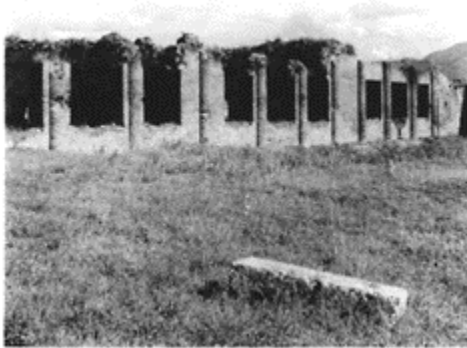
641 Western façade of the Central Baths at Pompeii. Begun after 62, these baths with their numerous large openings would have been well lit, in great contrast to the previous establishments which were enclosed and dark. This included the caldarium (the three windows on the right). This structure remained unfinished, but it would have had glass panels.
