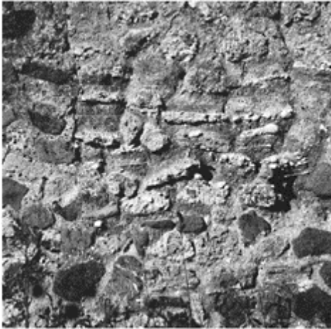
366 Pompeii, restoration of a wall after the earthquake of 62. Among the reused material are pieces of opus signinum paving (VI, 7, 2).
