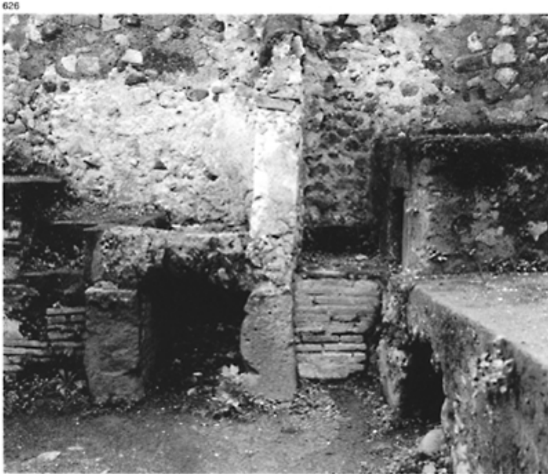
626 The kitchen of the Villa of Diomedes at Pompeii. On the right is the working surface where the fires were lit, with a small oven at the back. In the back wall is the mouth of the
