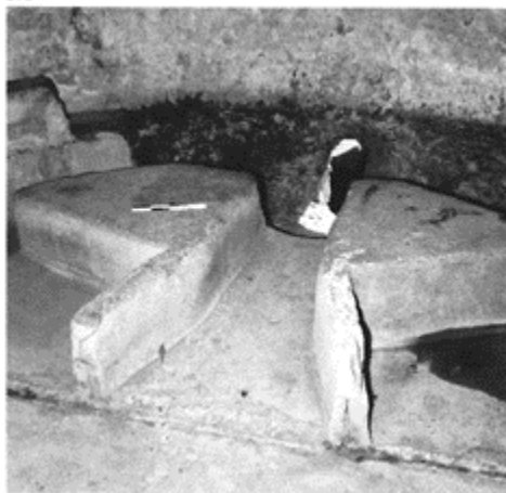
578 Division of the water into three channels in the castellum aquae at Pompeii. In front of the triple divider is the housing of the lead plate which once formed a dam for the water to
