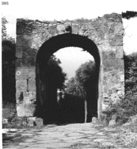
385 The Nolan Gate in the north-eastern section of the wall of Pompeii, made of blocks of tufa with dry
