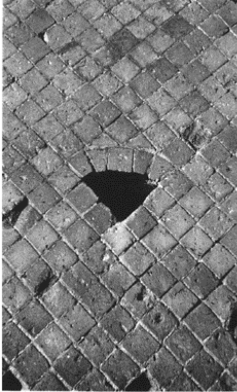
189 Detail of a particularly carefully made putlog hole in a fine reticulate facing. Pompeii VIII, 2, 14, c. 70.
