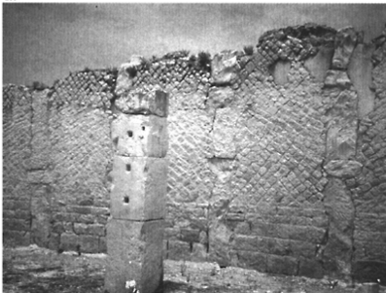
280 Building at Bulla Regia (Tunisia) with reticulated facings between vertical chains.
