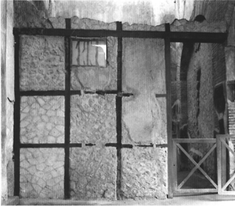
282 Herculaneum: timber—frame partition, opus craticium , built between 62 and 79 at the College of the Augustales. The infill is opus incertum and the whole was rendered. Thickness with rendering: 18cm. Section of the pieces of wood: 9×9cm.
