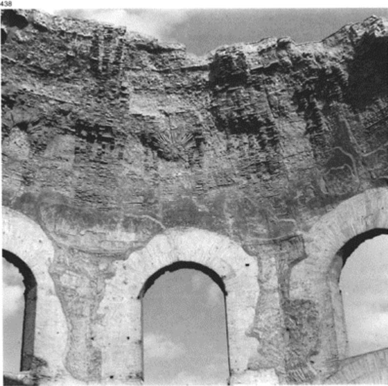
438 The interior of the dome of the 'Temple of Minerva Medica' in Rome. The transition from a tensiled to a circular shape is carried out by means of a progressive and undetectable tapering of the masonry. The structure is that of coffers and ribbing, defined by brick frameworks containing a fill of rubble. Notice that the strong ribs radiating out distribute the pressures
