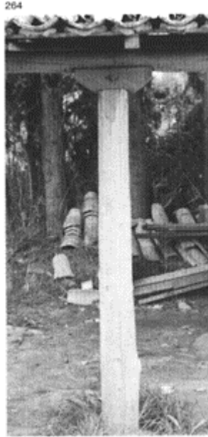
264 Technical perfection and the genesis of the capital in a rustic building in the Peloponnese.
