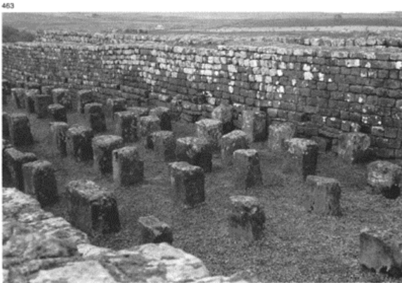
463 Hadrian's Wall: horrea of the garrison of Borovicus (Housesteads). Sockets and small supporting columns for the floor joists.
