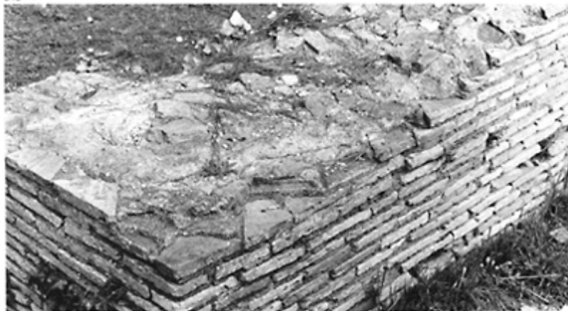
348 Masonry wall faced with triangular bricks. Ostia, beginning of the second century.
