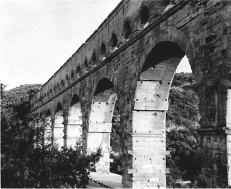
420 The middle series of arches in the Pont du Gard, showing the projections for supporting the centring and the three parallel rows of voussoirs; c. AD 15.
