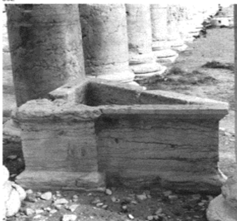
602 The basin of a triangular fountain, cut out of a single limestone block—an
