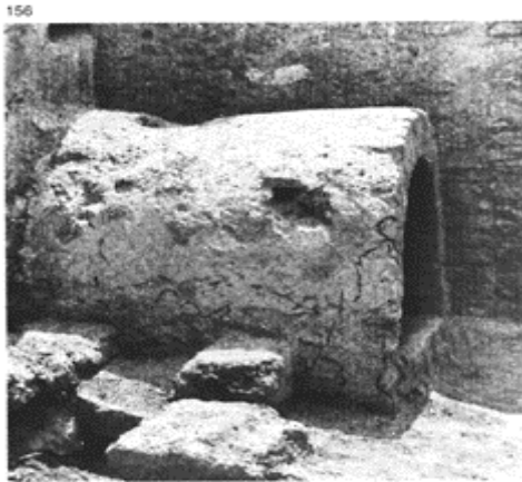
156 Temporary lime-kiln situated in a little garden of the House of the Iliac Chapel at Pompeii (I, 6, 4). (Photo: V. Spinazzola.)
