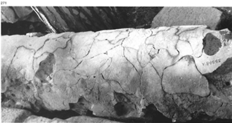
271 Column shaft of artificial polychrome marble. Fragments of different types were added to the column, placed in the cavities and fixed with the help of an iron cramp sealed with lead. Found in the marble depot of the port of Ostia.
