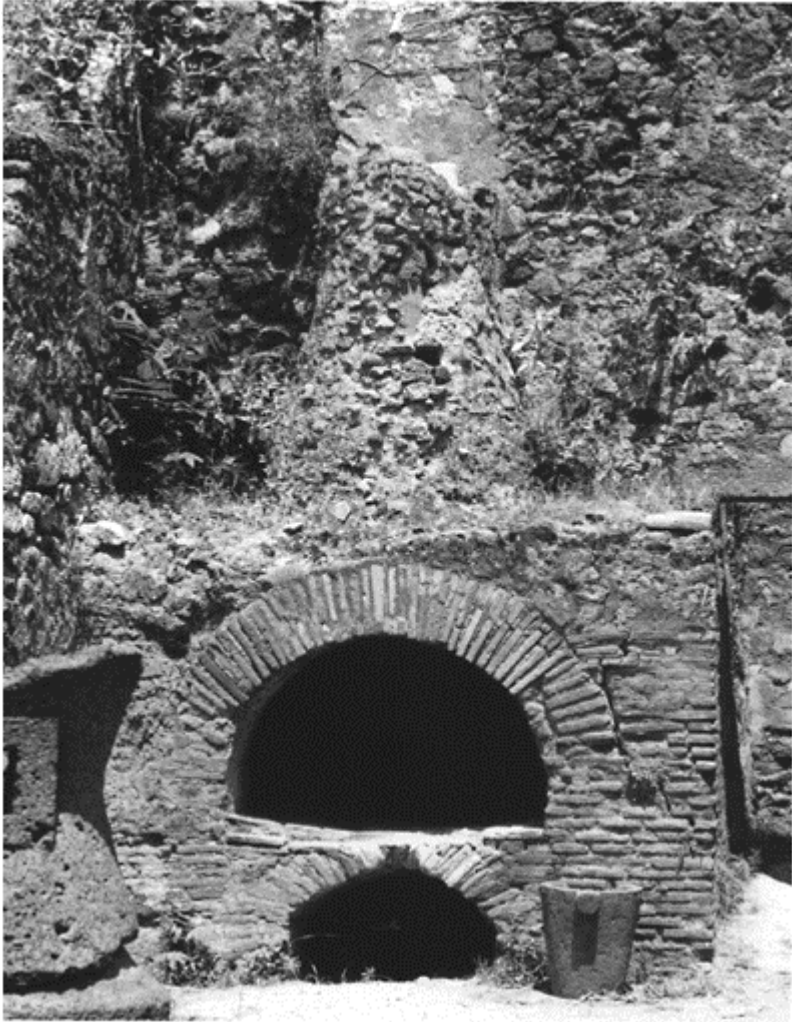
623 A baker's oven at Pompeii (VI, 2, 6). The chimney has a terracotta flue buried in the masonry; this arrangement could clearly also be used for heating, although that purpose is not found here.
