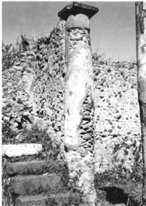
374 Masonry column made of rendered rubble stones of lava. The block of the capital is tufa. Pompeii, VIII, 3, 27.
