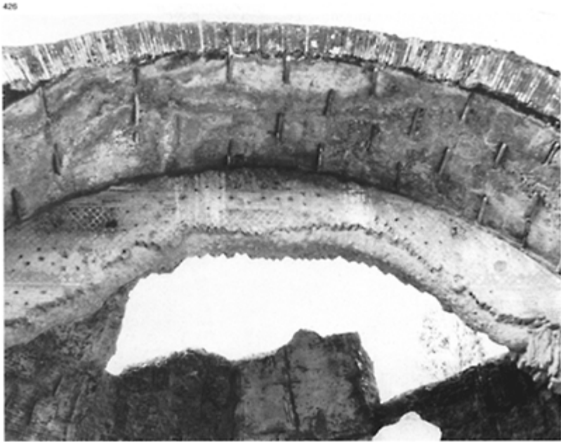
426 Marks of bricks placed straight on to the centring (which has collapsed) and ends of the radiating bricks visible in the intrados of the arch in the frigidarium of the Great Baths of Hadrian's Villa. Between 118 and 125.
