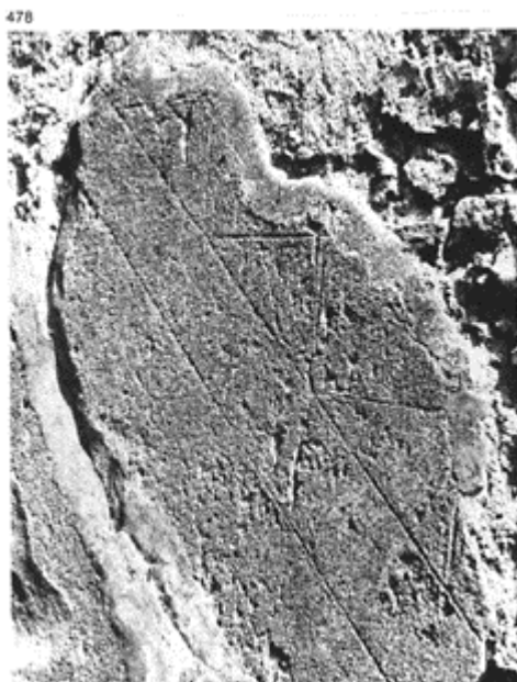
478 Preparatory marking, incised in the mortar, for a flight of wooden steps.
