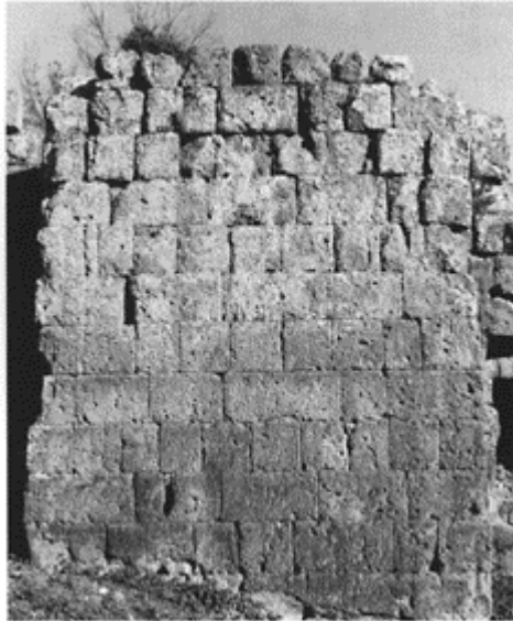
249 Facing of a tower on the walls of Falerii Novi, built after 241 BC with
