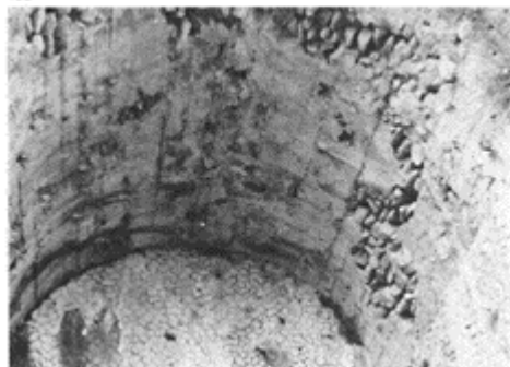
433 The traces of the planks or shutters of the centring in the intrados of an arch in the terrace at Terracina. Beginning of the first century BC.
