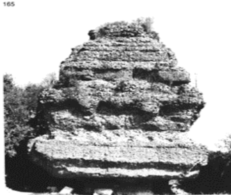
165 A large mausoleum on the via Appia which has completely lost its facings and is hollowed out, especially at its base, where rooms of a surrounding medieval construction,
