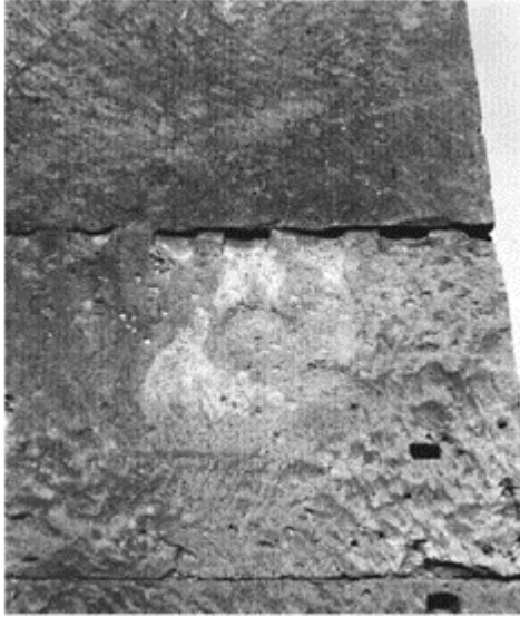
38 A block of tufa with the traces of the sockets for the wedges that were used in cutting it up (Pompeii VIII, 5, 30).
