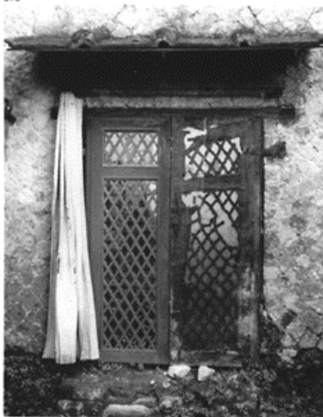
676 A door with double lattice leaves at Herculaneum (Eastern Insula II). The left-hand door is modern.
