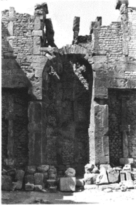
279 Thugga (Dougga), the Capitol (Antoninus Pius). A wall with niches, made of opus africanum with infill of coursed rubble bonded with mortar.
