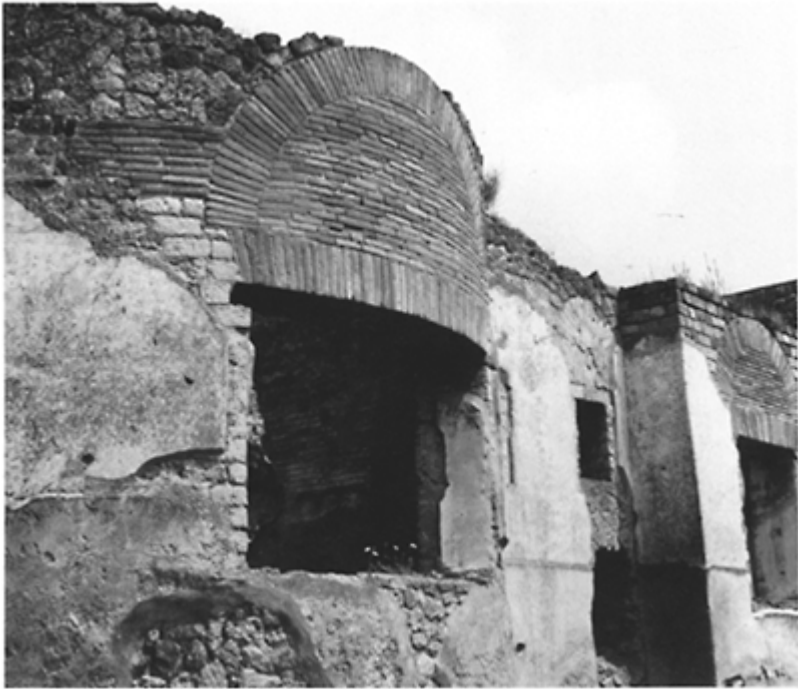
415 A window in an exedra of the Villa of the Mysteries. The flat arch serves as a lintel, and the relieving arch of bricks follows the circular shape of the wall.
