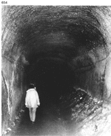
654 The 'grotto of the Sibyl'—a tunnel dug into the volcanic tufa in the Augustan period, between Lake Lucrino and Lake Averno. This allowed a rapid passage for pedestrians and vehicles between the facilities at these two stretches of water, themselves connected with each other and with the sea by an enormous canal, now filled in. Length of the tunnel:
