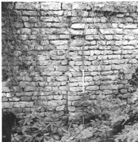
322 Facing of 'petit appareil' of the amphitheatre of Senlis (first century). The coarseness of the masonry of the facing is visible in the irregular size of
