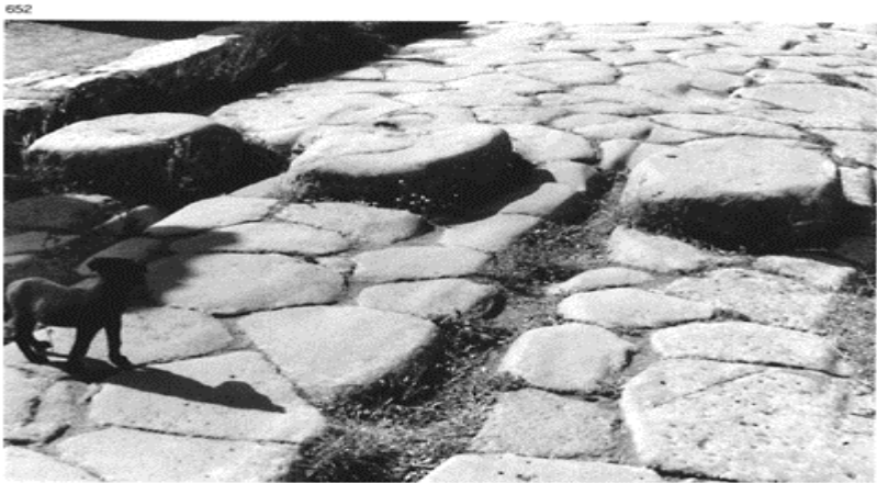
652 Detail of the via della Fortuna at Pompeii. The main streets of the city were paved with lava and edged by pavements. The lack of a sewer network to drain rainwater, household water and the water from fountains from the streets, meant that they could only be used by beasts of burden or
