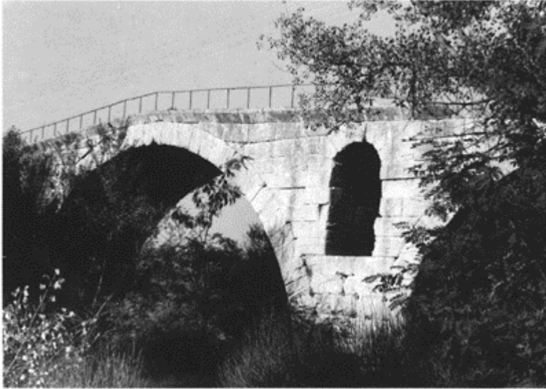
659 The Pont Julien, over the Coulon, near Apt (Vaucluse); 68m long, it has preserved its three arches (here the central arch and the hog's back are visible); each pillar has a flood-opening through it. Augustan period.
