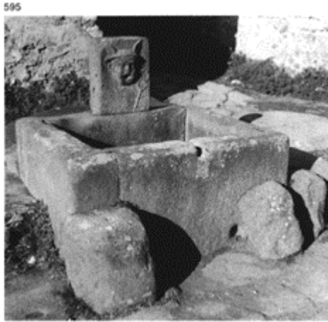
595 A public fountain at Pompeii, decorated with a head of Mercury. The supply pipe came out of the figure's mouth. The overflow channel is visible on the top of the rim, and, at a lower level, the outflow of the drainage hole VI, 8.
