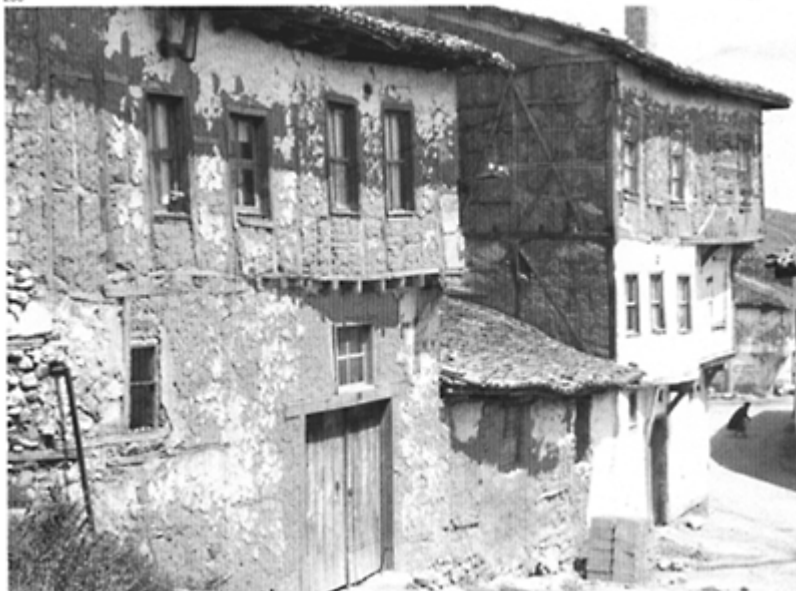
286 Timber-framed houses with corbelling, probably identical to ancient examples, in the region of Bursa, Turkey.
