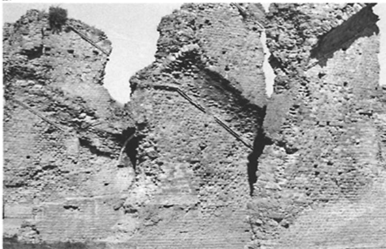
321 Amphitheatre of Fréjus (first century) built of 'petit appareil' in masonry with regular courses.
