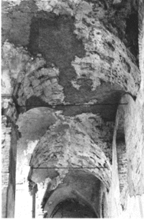
458 Rows of groined vaults made of masonry constructed on a permanent centring of square bricks. Ostia, House of Serapis.
