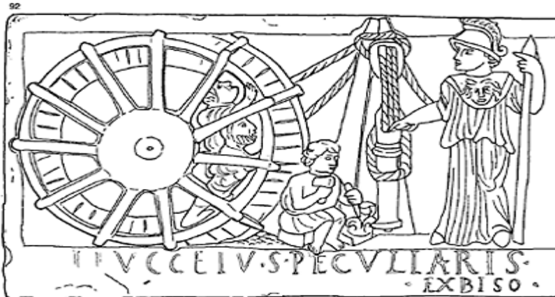
92 A lifting machine shown on a relief found at Capua. The motor wheel, operated by two workmen, is shown as independent from the crane, which is lifting a monolithic column into place using a block and tackle. The workman in the front is carving a capital.
