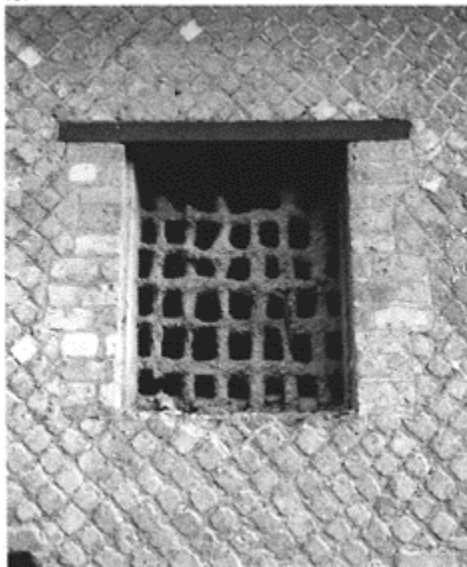
701 When ground-floor windows were of some size they were barred with an iron grille. This example is on the cardo IV, insula 5 , at Herculaneum.
