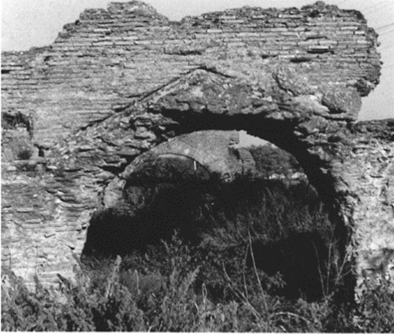
490 Remains of the roof support of an arched room in the Villa dei Sette Bassi. There were no timbers here—the tiles were placed on a sloping bed of mortar.
