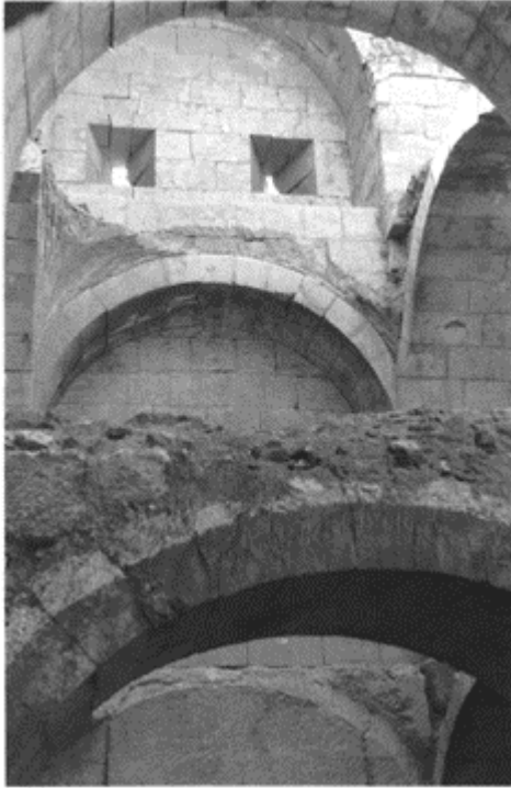
462 Halabiye (Zenobia), Syria: three successive vaulted levels of the ' Praetorium ' of Justinian, with arches built of stone blocks and groined vaults made of brick.
