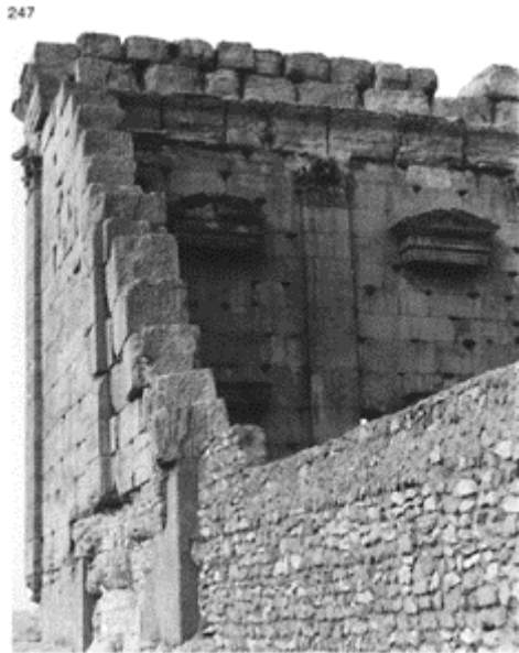
247 Wall made up exclusively of bonding blocks: peribolos of the Temple of Bel at Palmyra; first century
