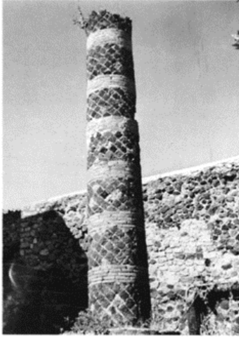
375 Masonry column alternating a tufa and lava reticulate and rings of bricks. Standing behind the Forum Baths at Pompeii, it carried a sun dial.
