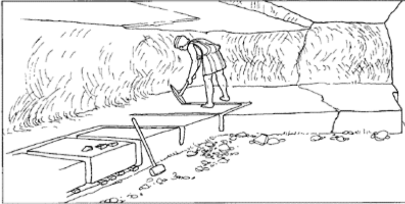
30 Reconstruction of quarrying in galleries in the tufa of Grotta Oscura (Latium).
