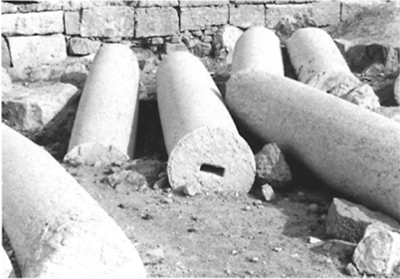
105 Monolithic column from the 'Camp of Diocletian' at Palmyra, with a lewis hole. Height: 4m; diameter: 55cm; lewis hole: 15×4cm.
