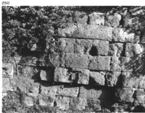
250 Ramp of the via Flaminia near the Civita Castellana. The courses of rectangular blocks of tufa follow the slope of the road with alternate rows of stretchers and rows of headers. Work began in 220BC.
