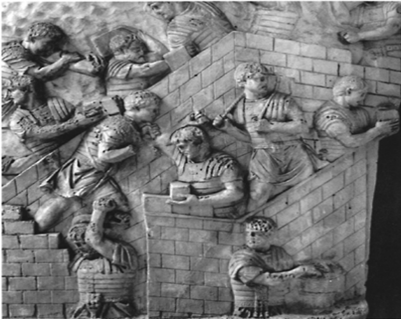
177 Legionaries building a fortification with unbaked bricks. Trajan's Column.
