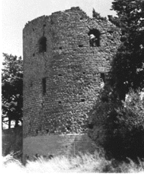
320 A tower in the walls of Fréjus faced with opus vittatum in which the putlog-holes are visible. Beginning of the first century AD.
