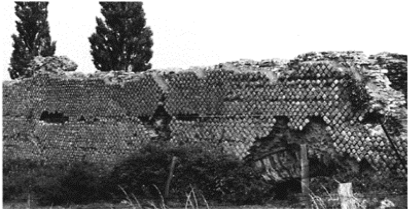
563 The aqueducts of Lyon, after crossing a depression almost parallel to the Rhône, using siphons, were for a short distance raised on sections of massive construction. The decrease in
