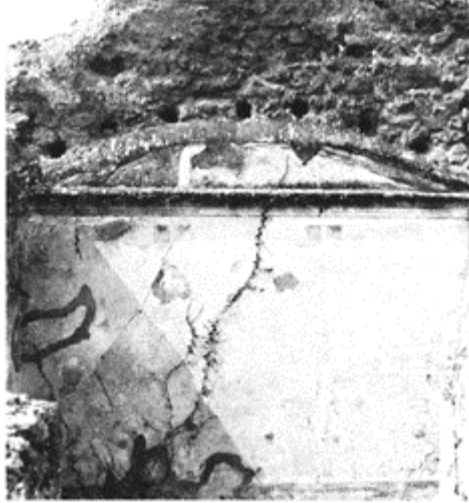
473 Remains of the sockets of the beams supporting a hanging vault, covering a room at Pompeii, IX, 5, 21.
