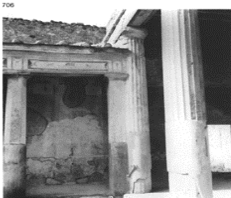
706 The so-called 'Rhodian' column, where two porticoes of different heights meet in the peristyle of the House of the Silver Wedding (V, 2, 1).
