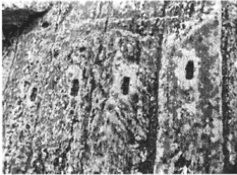
103 Lewis holes on the outer curve of the archstones of the ambulatory in the arena of Arles.
