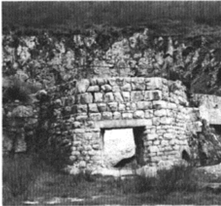
147 Lime-kiln situated right at the foot of the quarry supplying it at Itri, southern Latium.
