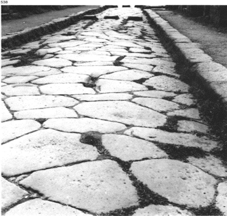
538 The paving of a commercial street in Pompeii, the via della Fortuna, of large slabs of lava, about 30cm thick.
