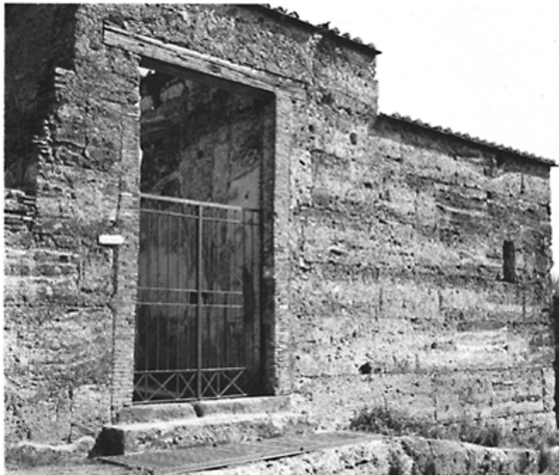
668 The House of the Surgeon, built in the fourth century BC with a frontage of limestone ashlar (VI, 1, 10).
