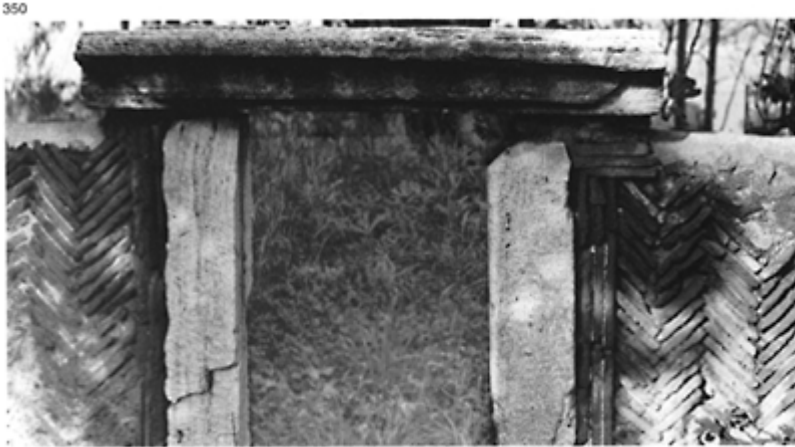
350 Ostia, tomb of the second century on the Isola Sacra with an unusual facing of bricks arranged in opus spicatum in the manner of a floor-covering.
