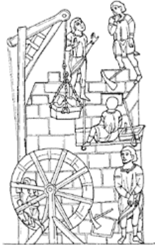
96 Medieval lifting machine, powered by a large wheel. ( Histoire Universelle , thirteenth century; JPA.)
