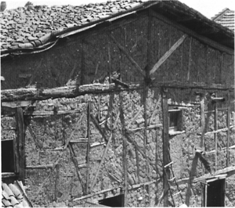
134 Timber framing with clay infilling in the traditional architecture of the region of Bursa (Turkey).
