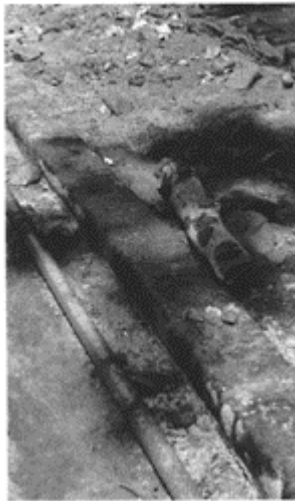
606 Temporary water supply network at Pompeii in December 1980.
