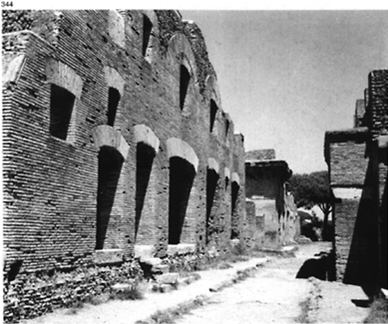
344 Street in the Insula of Diana at Ostia. The expansion of the city at the beginning of the second century saw the triumph of brick in the majority of façades. In the foreground the 'Casa dei Dipinti'.
