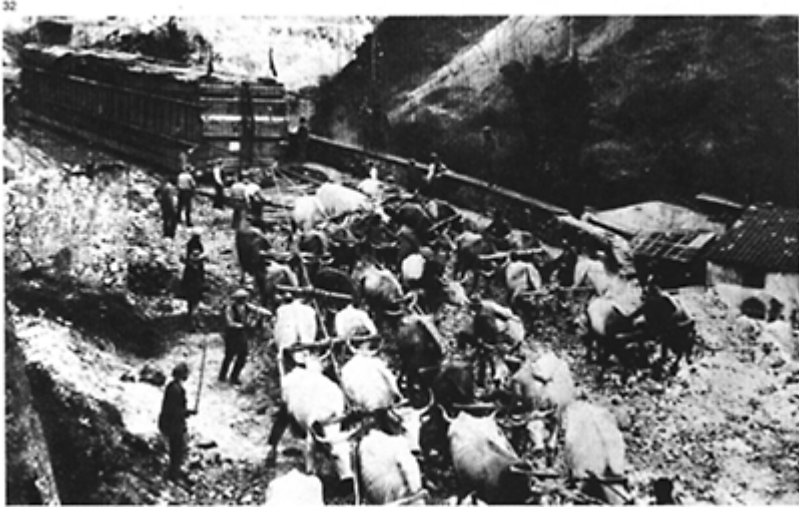
32 Mussolini's monolith being transported on a sledge, pulled by a team of sixty oxen, Carrara, 1928. (Photo: Hrand.)
