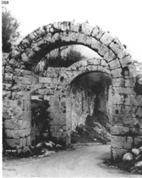
388 The Porta Maggiore at Ferentino ( Ferentinum ). The two arches of an opening 4.2m wide with a double row of short voussoirs are to be compared with the outflow of the Cloaca Maxima ; date around 80BC.
