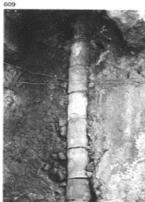
609 Down-pipe from an upstairs latrine in a modern farm at Pompeii.
