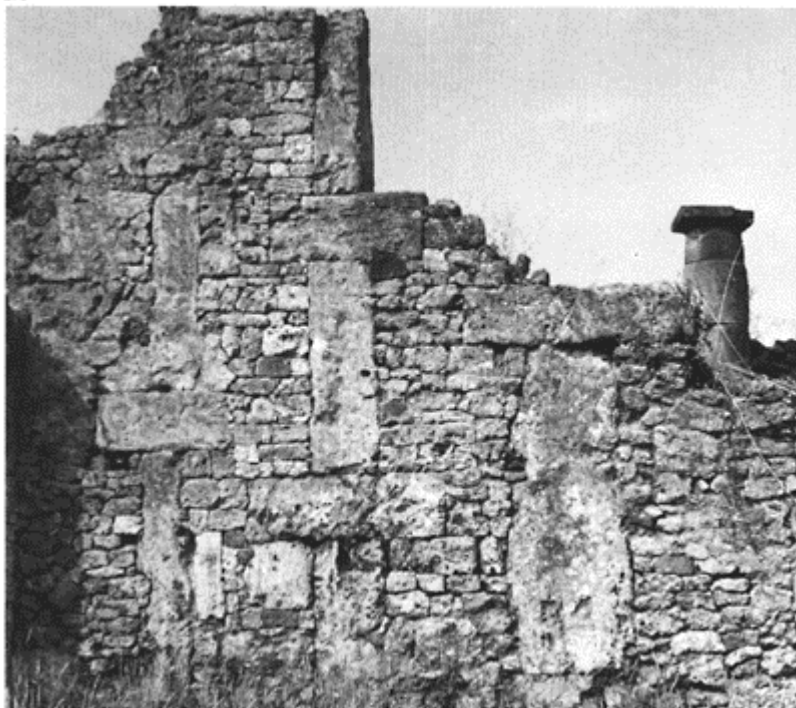
276 Wall of ' opera a telaio ', opus africanum , at Pompeii, in a house of the first Samnite period, made of Sarno limestone (VII, 3, 16).
