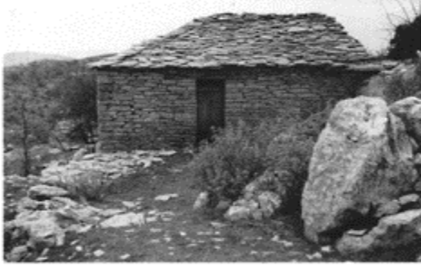
503 Roof covering of limestone tiles on a rural building in the Peloponnese.
