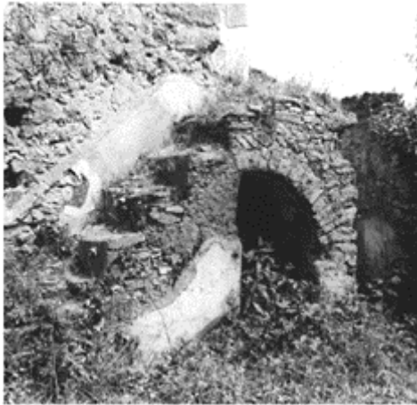
720 Stairway made of masonry in V, 2, d. The supporting piers were relieved by one or more vaults and used for storing various things.
