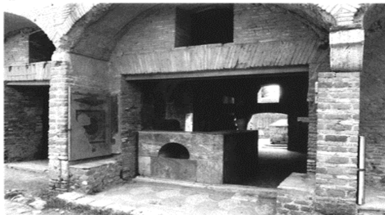
732 Shop-front of a thermopolium in the street of the House of Diana at
