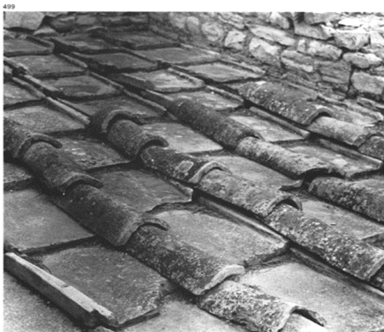
499 An ancient roof with flat flanged tiles ( tegulae ) and junction-covers ( imbrices ) reconstructed at Vaison-la-Romaine.
