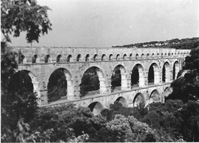
560 The Pont du Gard. The facings are made of large stone blocks up to the arches of the third level; the walls of the channel are of rubble masonry. Augustan period. Length: 275m; height: 48.77m.
