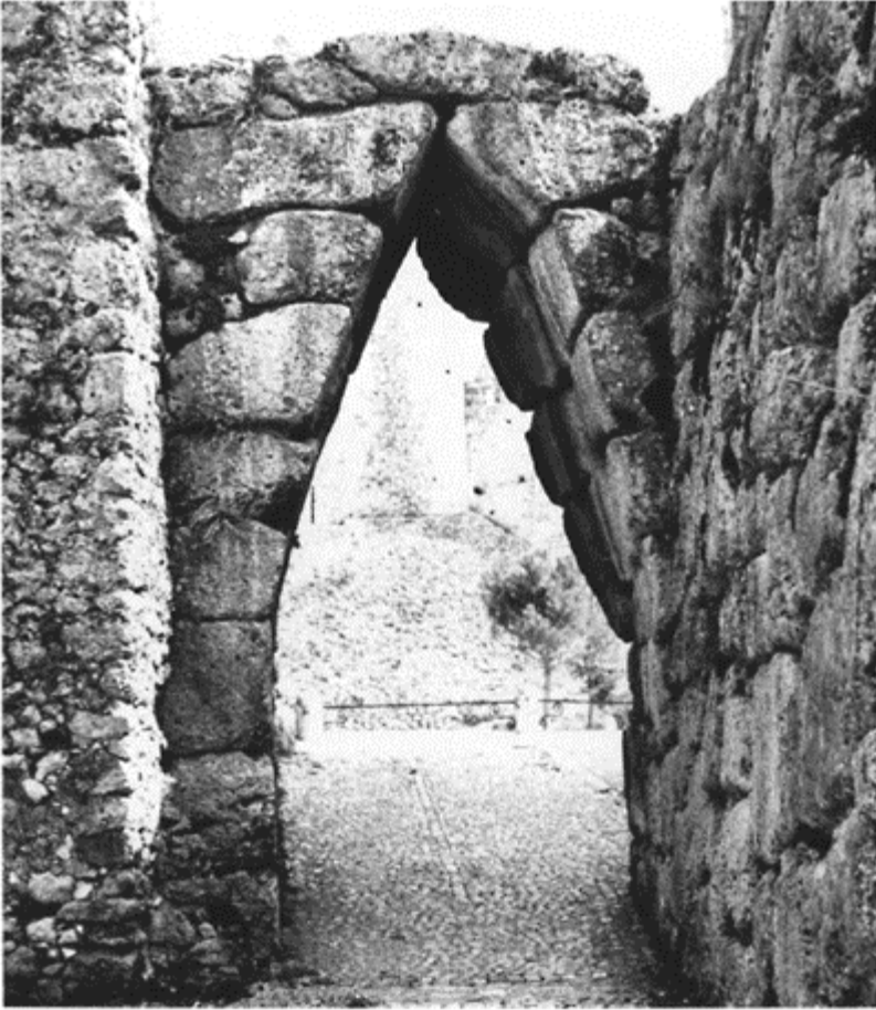
389 The great corbelled gate in the megalithic wall of Arpino (southern Latium) of polygonal stone, the so-called second type. Width: 1.9m; height of the opening: 4.2m. Fifth century BC.
