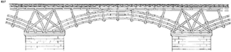
657 Reconstruction of the bridge over the Danube from the relief on Trajan's Column. (After A.Choisy.)
