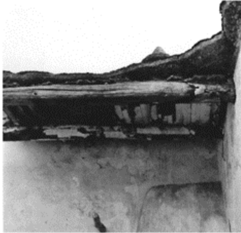
469 Ceiling of a ruined farm at Pompeii, showing the same structure as ancient ceilings: the beams support a parquet on which a layer of mortar is placed.
