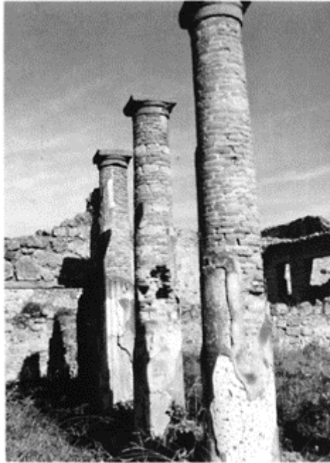
373 Masonry columns from a peristyle at Pompeii (VI, 13, 9): two are made of bricks, the third of opus mixtum ; the capitals are dressed tufa. Fluted stucco decorated the outside.
