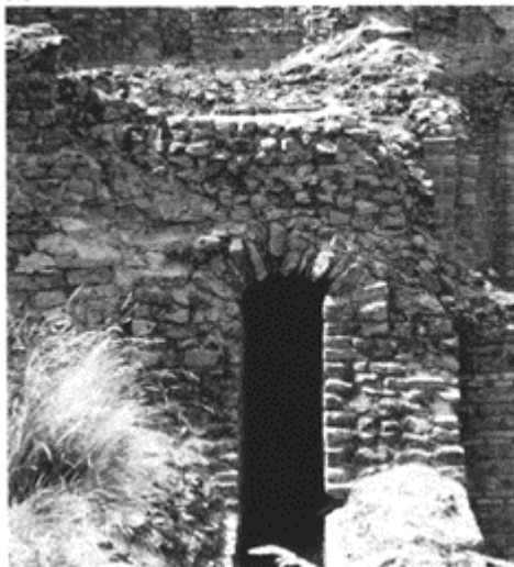
618 A tunnel separating the retaining wall, left , from the wall of the building, right , at the cryptoporticus of Bavay (Nord).
