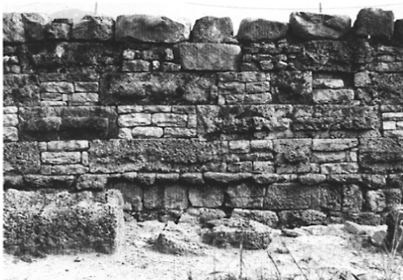
274 'Chequer-work' construction at Velia, with coursed rubble infilling. (Third century BC.)
