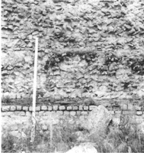
341 Rubble in reticulate arrangement in the walls of Bavay. End of the third century.
