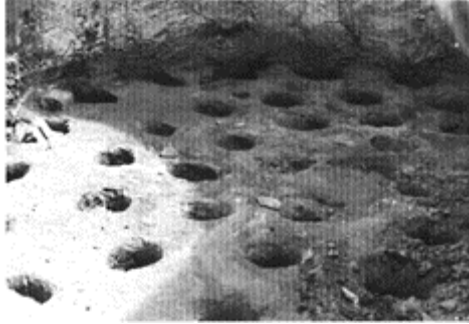
142 The internal plate or ledge of the same kiln as in fig. 141 and its heat holes or flues.
