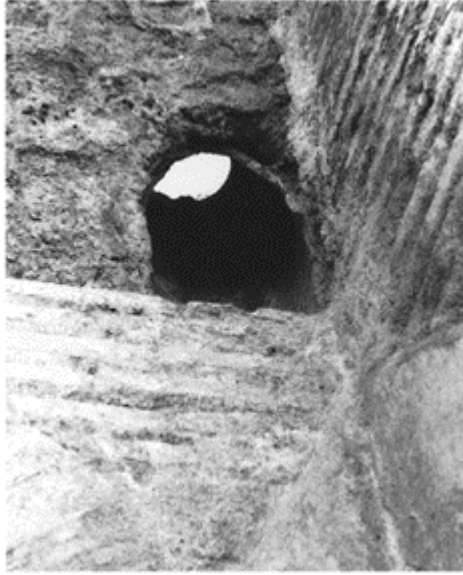
635 A chimney to remove smoke, linking the cavity of the double wall with an opening at the spring of the vault. Another chimney opened symmetrically in the opposite wall. Caldarium at the House of Julia Felix, Pompeii, II, 4.
