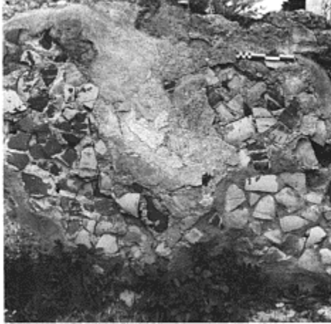
514 Ceramic fragments, intended to reinforce a wall rendering, first peristyle of the House of the Faun at Pompeii.
