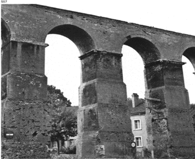
557 The arcaded section of the aqueduct at Metz ( Divodurum ) crossing the Moselle at Jouy-aux-Arches. First century.
