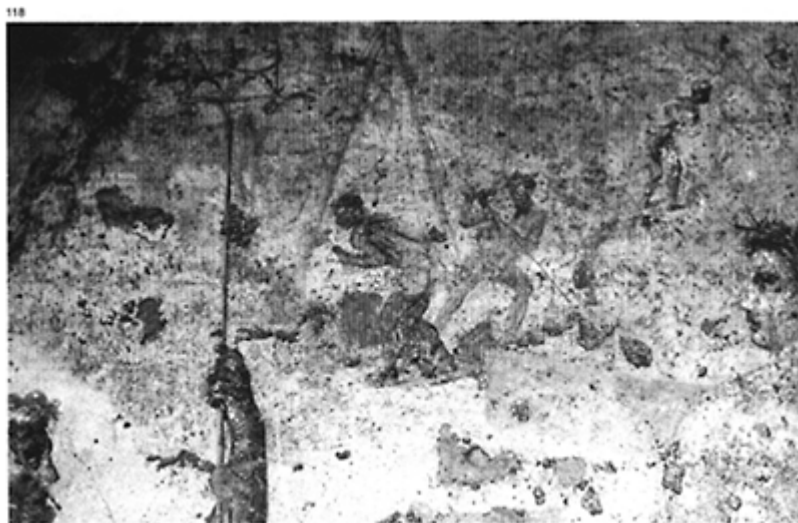
118 Painting from the House of Siricus showing a scene on a building site. Pompeii, VIII, 5, 26–57.
