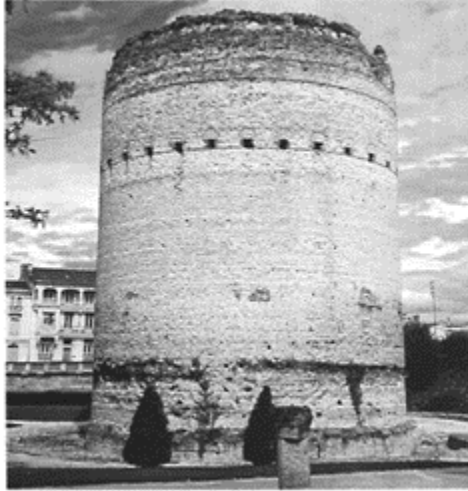
338 The ‘Tour de Vésone’ at Périgueux, a large fanum with circular cella, erected at the earliest in the reign of Trajan, is one of the first Gallo-Roman monuments to use brick.
