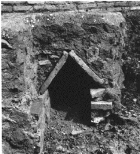
615 Section through a drain at Ostia with a gabled cover made of slabs.
