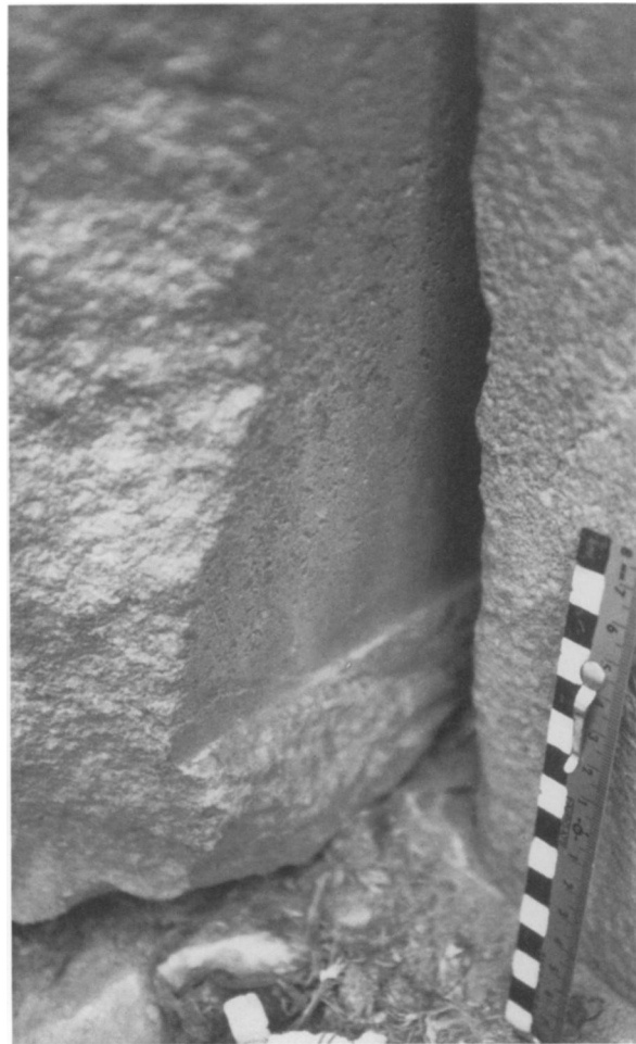
Fig. 9. Joint showing sawn area on in situ block.
