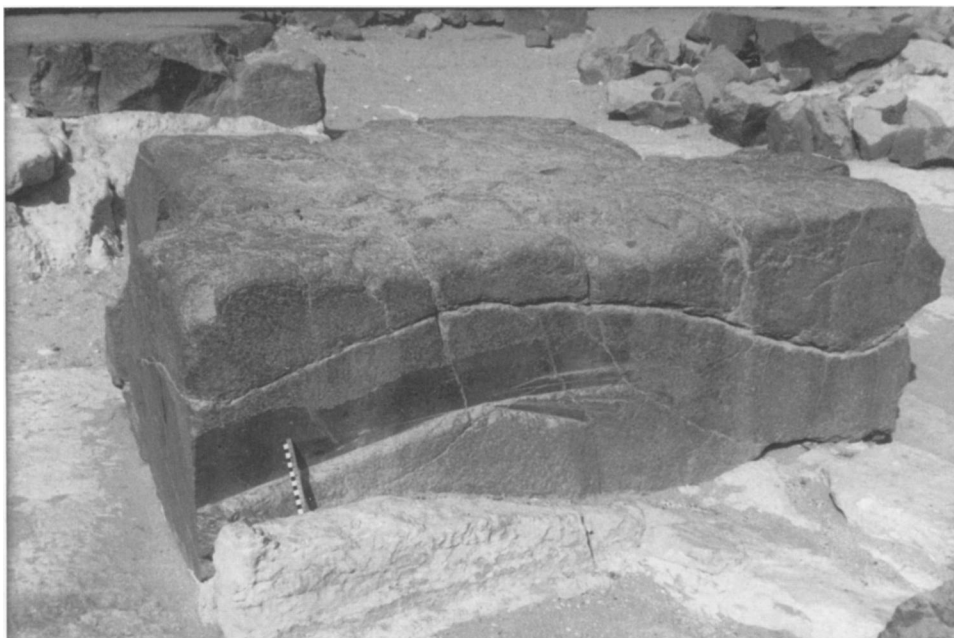
Fig. 2. Block A, from east.
