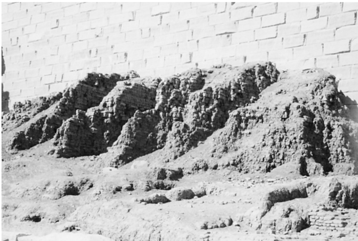
Figure 7.19 Remains of a mud brick ramp in the Karnak temple, Luxor
