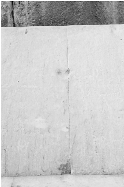
Figure 7.7 A rising joint between two large casing-blocks in the Great Pyramid
