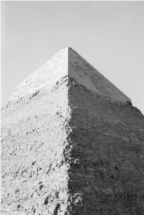
Figure 7.15 Precisely fitted casing-blocks at the top of Khafre's pyramid at Giza
