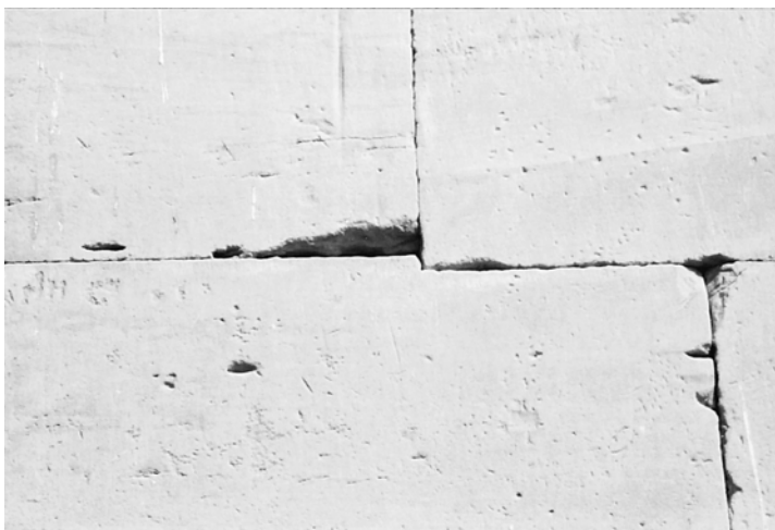
Figure 7.14 Large stone blocks were made to fit adjacent blocks
